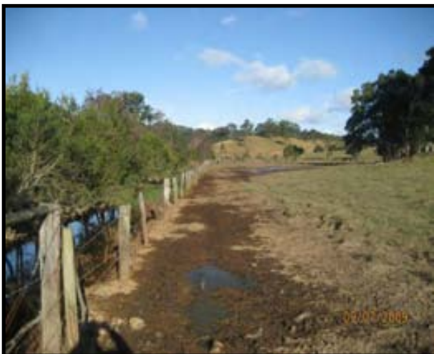
Before: Blacks drain 1500mm x1500mm (average) showing chronic signs of acidity such as scalded pastures and drain water pH < 3.5
