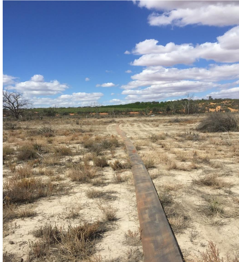
(b) 200-long lay flat hose to convey water to the basin
