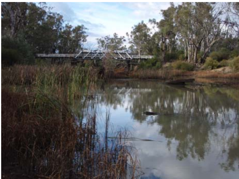
Figure 8-138. Site 4, Gee Gee Bridge (upstream view).
