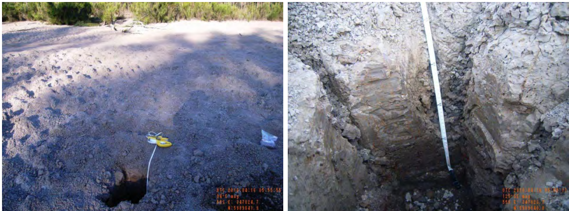
Figure 7 – Photographs of site 40383_5, showing the mid stream channel surface condition and the shallow soil profile of very dark brown, strong, silty clay loam and clay.
