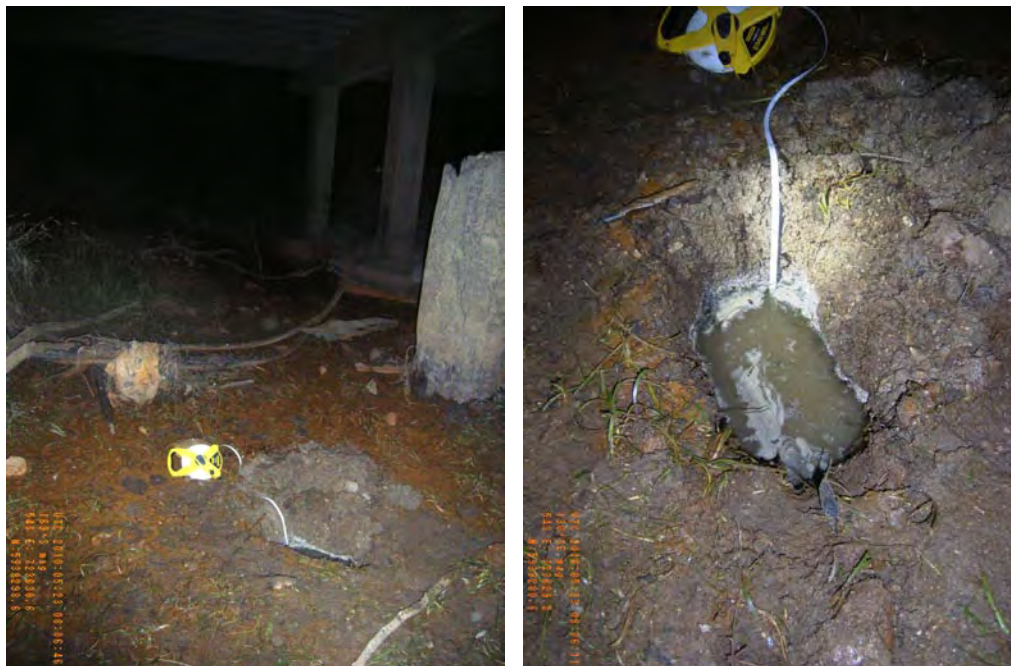
Figure 4 – Photographs of site 40851_2, showing the surface condition and the soil profile of very soft, dark yellowish brown sandy clay loam overlying very weak, dark greyish brown silty and clay loam sandy.
